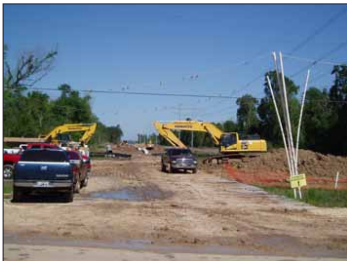
The Keystone XL Pipeline under construction in SE Texas.
